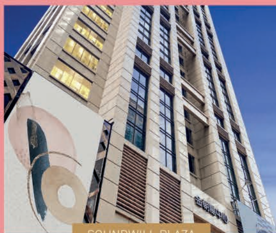
SOUNDWILL PLAZA COMMERCIAL CAUSEWAY BAY
